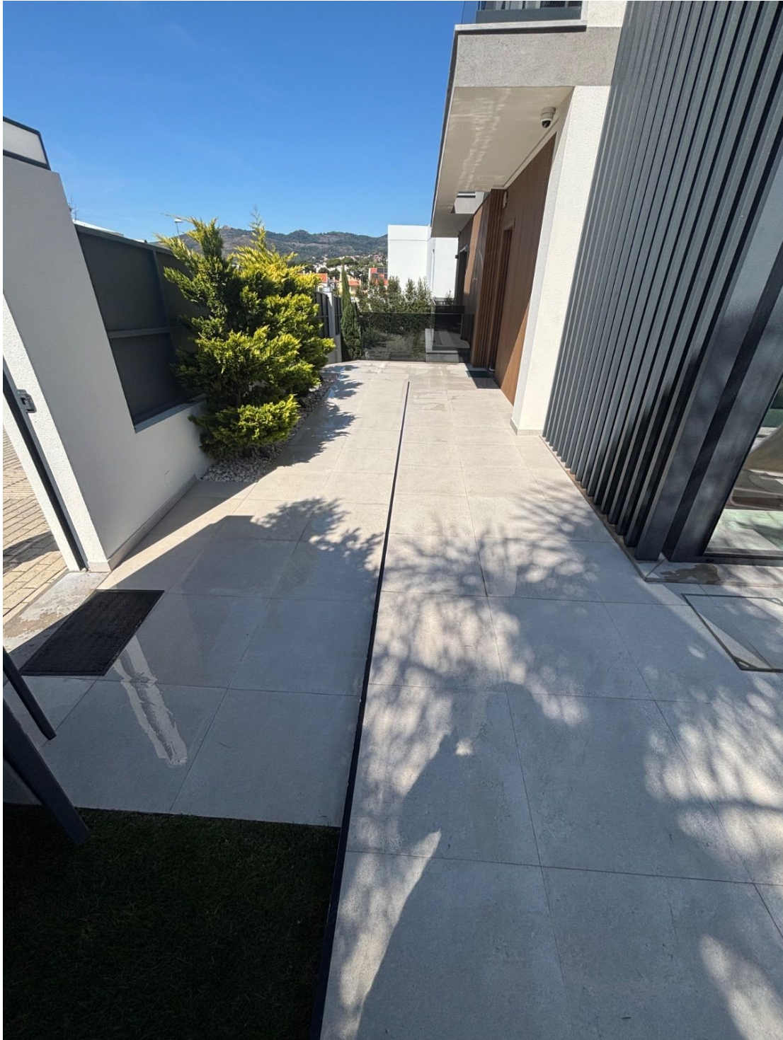
Exterior paving and drainage
